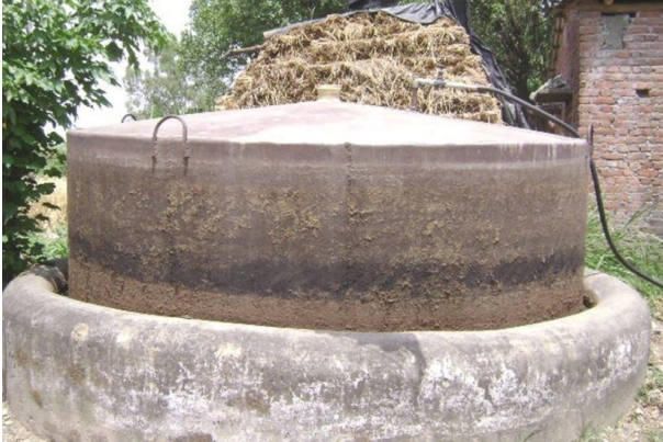
A View of Biogas Plant
